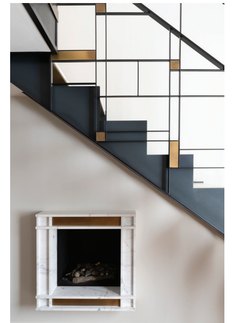
A new stairway leading from the kitchen to a service area, designed by 8&A architetti in black iron with brass inserts.
